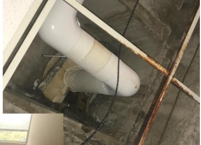
Damaged plumbing pipe leaking water (upper right)
