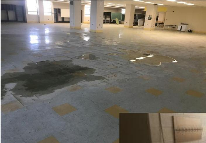
Settled water from roof leakage(upper left)
