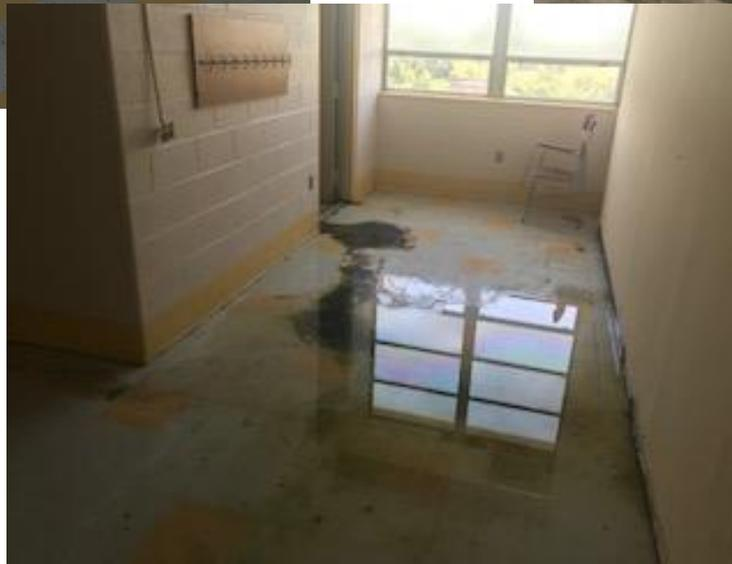
Settled water from roof leakage near stairwell (middle)
